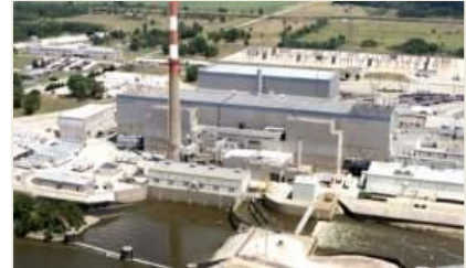
Exelon's Quad Cities Generating Station is a two-unit boiling water reactor (BWR) plant located in Cordova, Illinois (USA).
