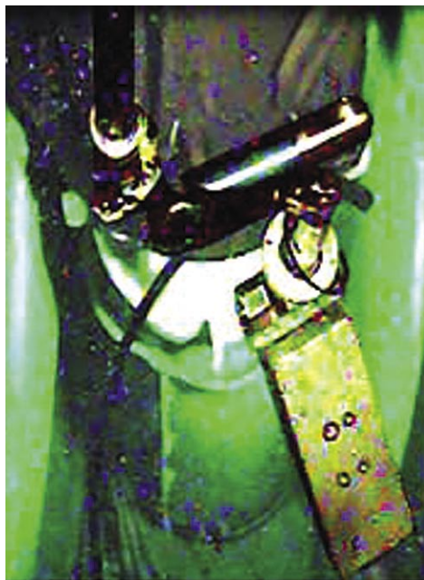
An NM200UW (lower right) deployed within the belt-line area of the jet pump of a BWR. Image distortion in the photo is due to high radiation.**
